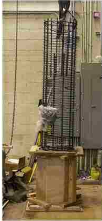
a). Column reinforcement
