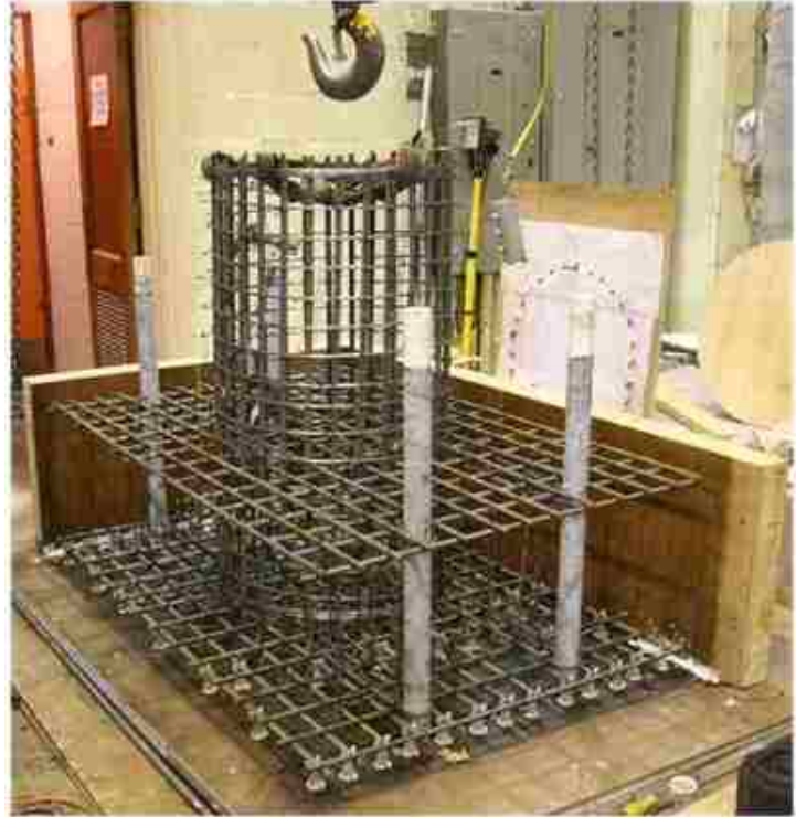
b). Shaft-Footing reinforcement
