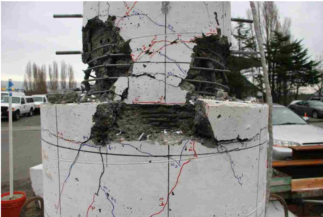
Figure C-0-6. DS-1 – Column damage after cyclic testing
